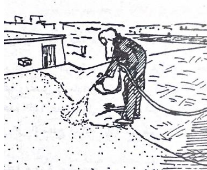
Figure. (4-D) : A layer of insulating material for concrete surfaces spread by a spray device
